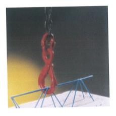
Our wide slabs are provided with under-reinforcement, with a flat and smooth surface on the underside. After placing the wide slabs the pipework is laid and the upper reinforcement applied.
